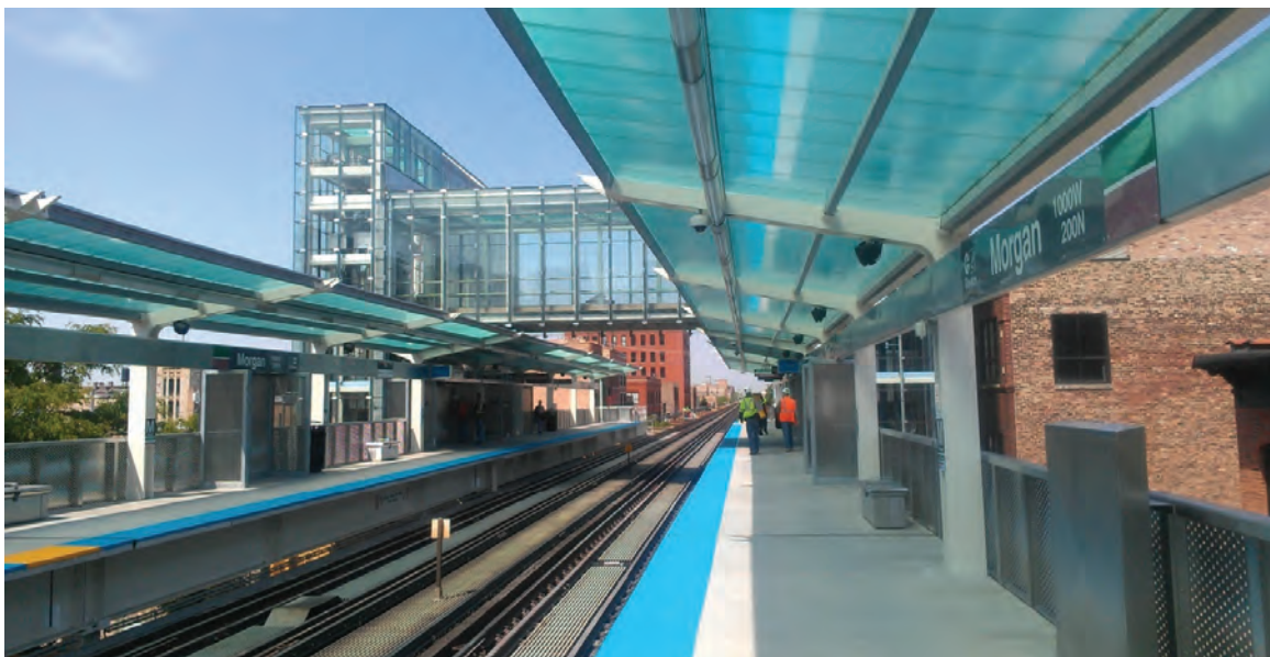
Figure 2: The new Morgan Station on the Chicago Transit Authority Green Line, which opened in 2012. Source: chicagotribune.com
